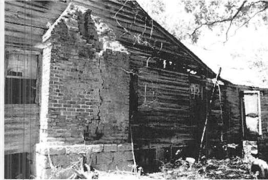
West end on left (Furman barracks). East end below shows clapboarding over log and deteriorated rear shed room and kitchen ell in far right.
