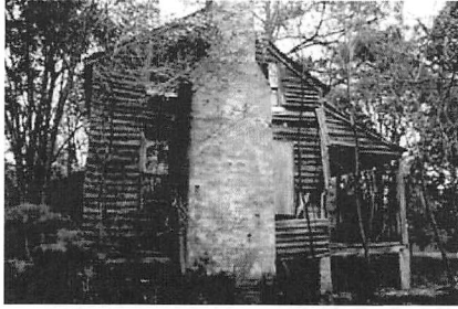
West end on left (Furman barracks). East end below shows clapboarding over log and deteriorated rear shed room and kitchen ell in far right.
